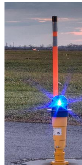
Figure 4-1. Example of Snow Pole Installed on Taxiway Light.
