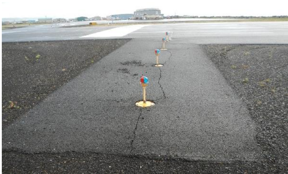
Figure 2-1. Unalakleet Runway Threshold End Lights (Photograph by Shawn Crites).
