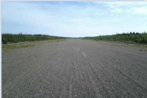
Gravel surfaces are common at most community and local NPIAS airports
