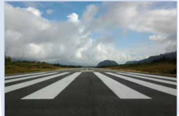
Airfield surface conditions will be remeasured
