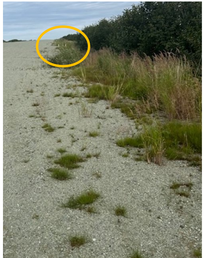
Figure 15. Encroaching Vegetation is Obscuring Edge Lights at Tuntutuliak (A61). The yellow oval photograph indicates the location of the lights.
