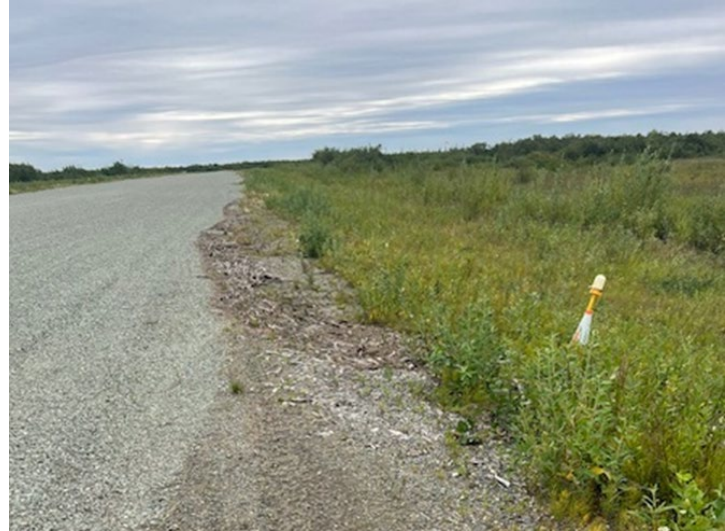
Figure 11. Debris Inside the Light Line of the Runway at PKA.
