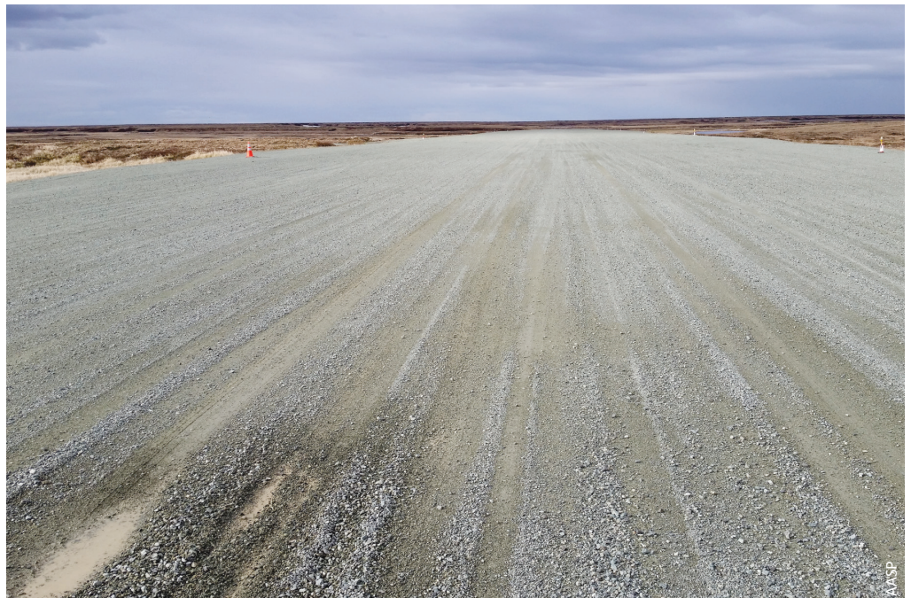
Rutting seen in 2023 during a 5010 inspection at Kongiganak Airport, one of the airports considered in the AASP Western Alaska Airports Resiliency Study.
