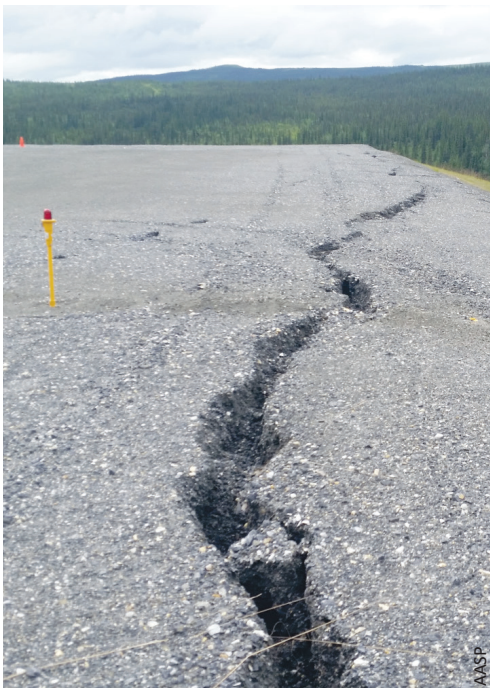
Longitudinal cracking seen in 2023 during a 5010 inspection at Kiana Airport, one of the airports considered in the AASP Western Alaska Airports Resiliency Study.
