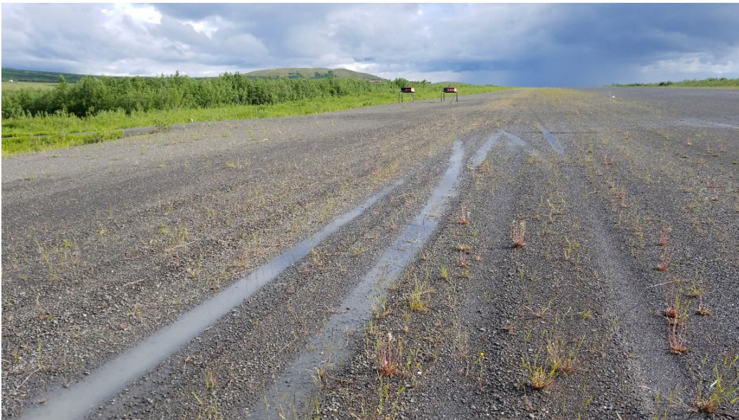
Figure 9. Rutting of the Runway Surface at St. Mary's (KSM) (Photograph taken by DOT&PF, 2021).
