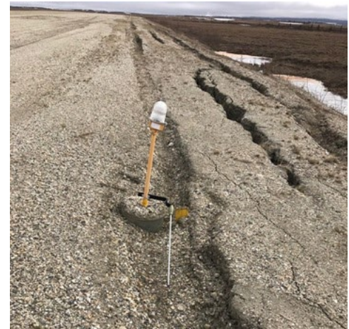
Figure 4. Shoulder Rolling Interfering With the Lighting System at Noorvik Airport (D76) [DOT&PF, 2019].
