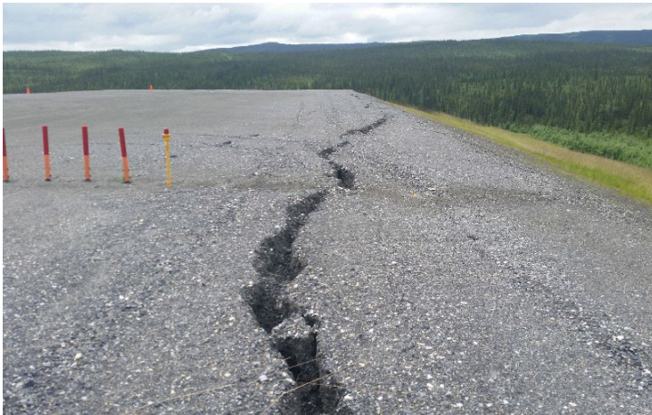
Figure 6. Longitudinal Cracking at Kiana Airport (IAN) [DOT&PF, 2023].
