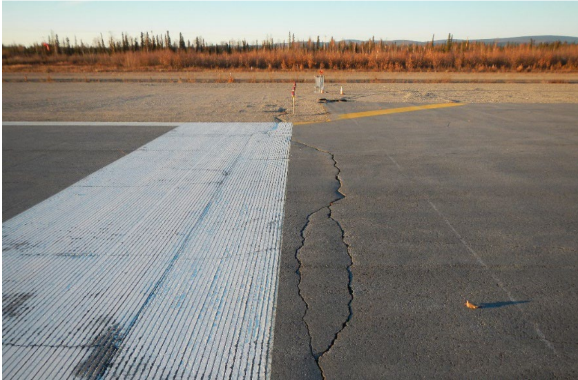
Figure 10. Northway Airport Runway
