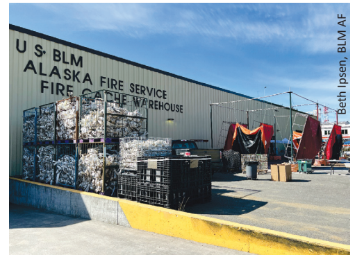
The BLM AFS Fire Cache Warehouse at Fort Wainwright, where fire equipment, gear, and supplies are stored.
