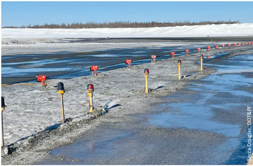
Threshold lights (orange), elevated runway end lights (red/green) and taxiway lights (blue) at Anchorage International.
