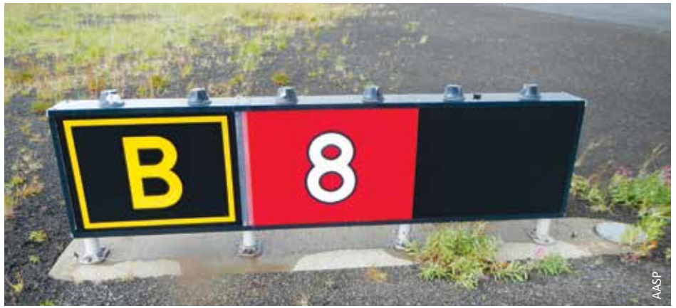
Airports with multiple runways feature lighted runway and taxiway signs to guide pilots, like this one in Unalakleet.
