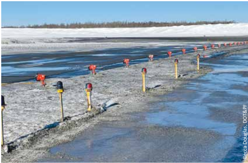
Threshold lights (orange), elevated runway end lights (red/green) and taxiway lights (blue) at Anchorage International.
