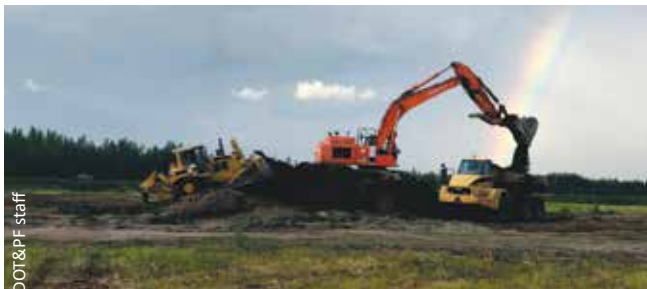
Galena airport 2018 reconstruction.
