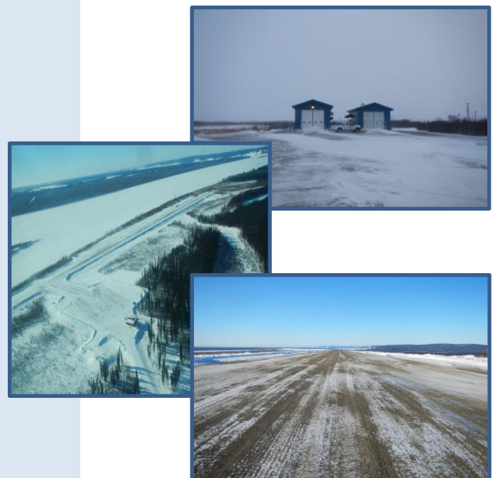
Left: Aerial of the Koyukuk Airport Top Right: SRE Buildings at the Napakiak Airport Bottom Right: Nulato Airport's Runway
