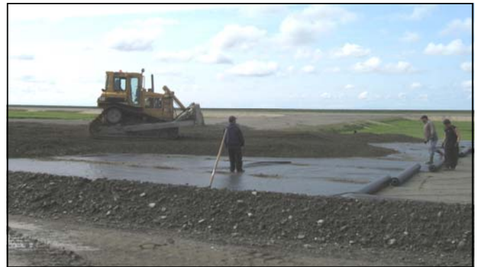
Placement of geotextile separation and sub base at a rural airport
