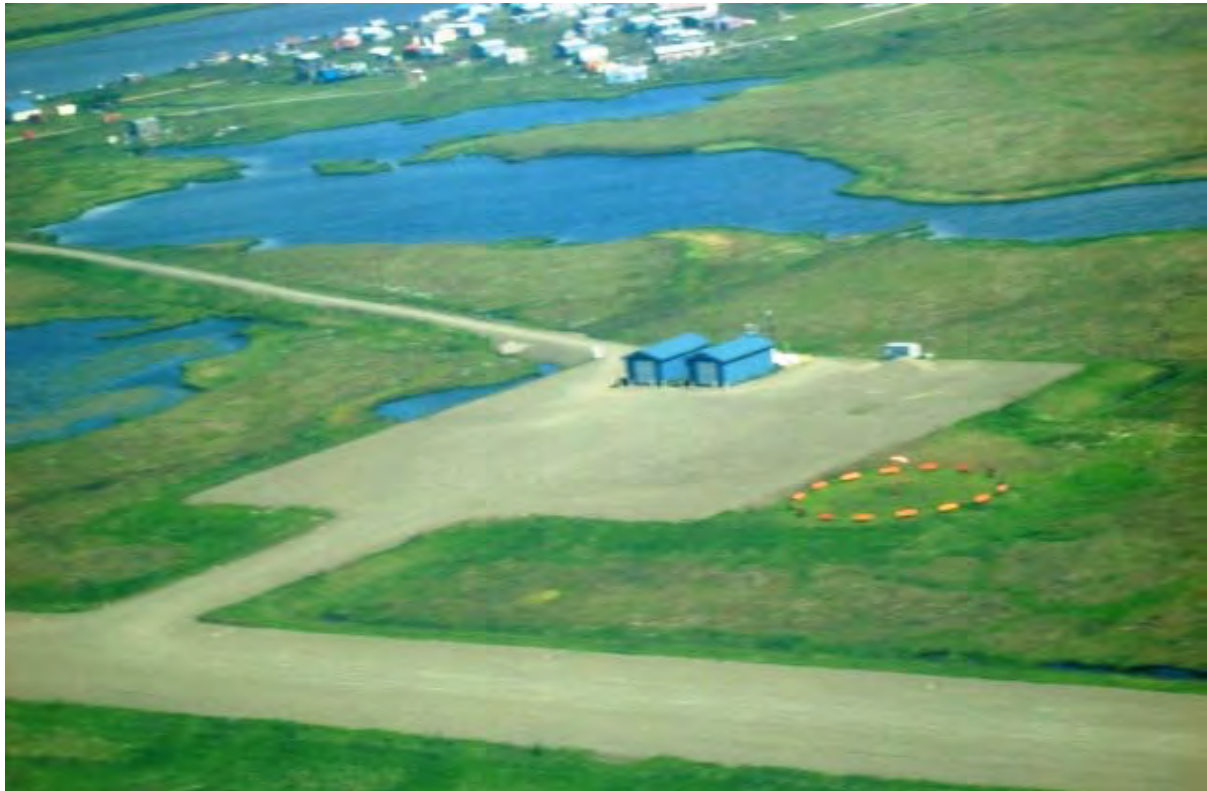
Figure 15. Facilities at Eek
